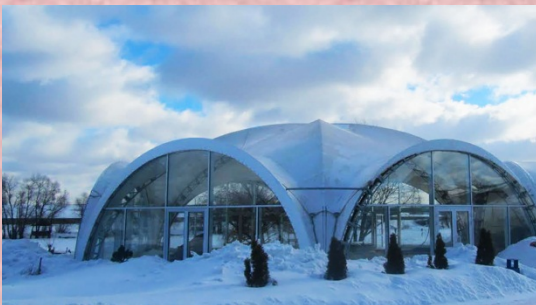
Restaurant tent, the leisure complex «Yudino Park»
